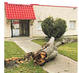
Fallen tree by Birkhead Hall.
