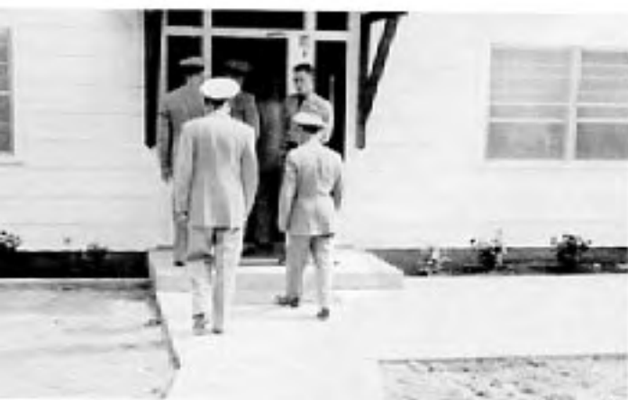
Inspection of Phelps Hall.
