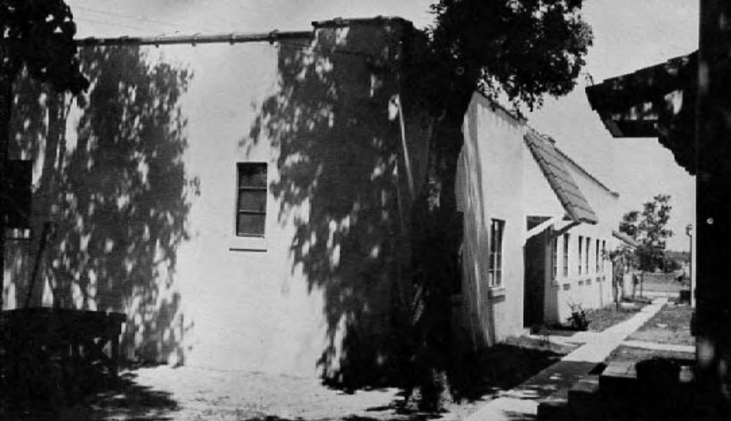
Armory Building and Theater
