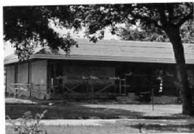
Library under construction.
